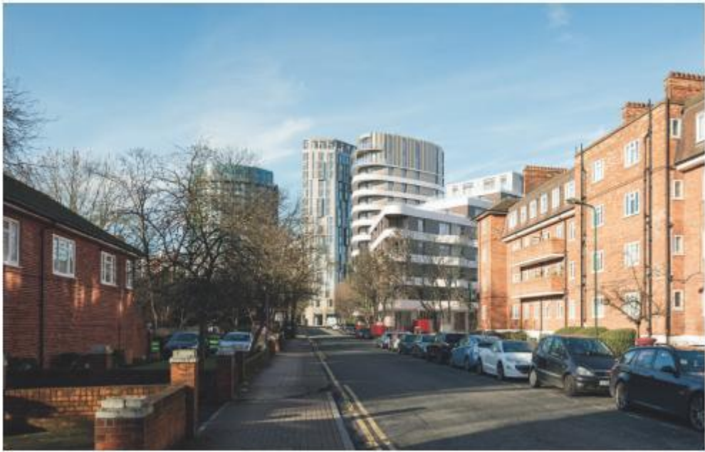
View West along North End Road
